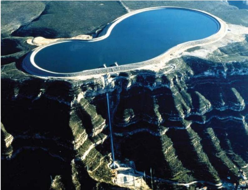
**2. Pumping up wind.** Spanish renewables giant Iberdrola's 1989-built 635-MW La Muela pumped storage facility will be followed by the 852-MW La Muela 2, slated to be operational in 2012. The ability to dispatch pumped storage power helps to mitigate the variability of wind power. *Courtesy: Iberdrola*
